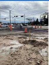
Cleaning & stripping paving forms from Loop 494 northside
