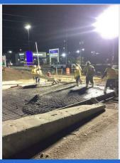
First truck deploying on north side of pour
