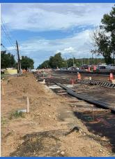
Setting paving forms along Loop 494 south side
