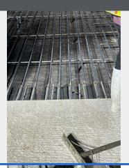
Longitudinal steel welded at start of paving pour #5
