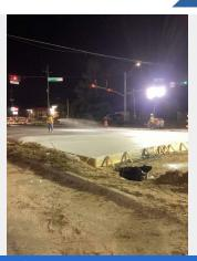
Applying curing agent to fast-track paving
