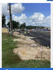
Setting paving forms along south end of Loop 494
