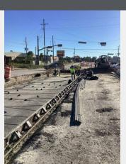
Clearing debris and prepping east end of paving pour #6
