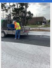
Primate Construction sealing joints in pavement
