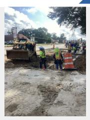
Cutting down subgrade and setting paving forms east of Kingwood Elite
