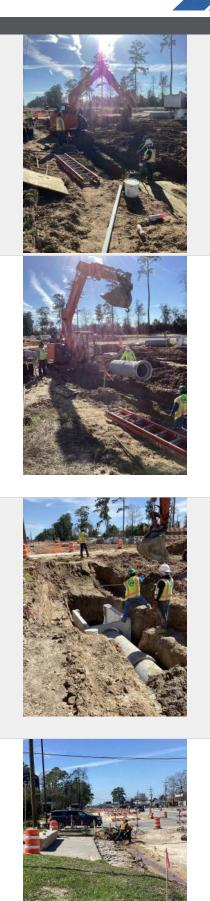
Go view the full size image Placing 24" RCP on run from C14 - C16
