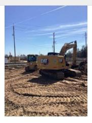
Backfilling C20/trenching for 30" RCP to C16 Q Latitude: 30.06844001, Longitude: -95.23932498
