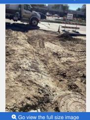
New Image2:15 pm 01/06/2025Latitude: 30.06857943, Longitude: -95.24208121HBC cut a small ditch from the roads edge to the manholeHarper Brothers ConstructionNorthpark Drive
